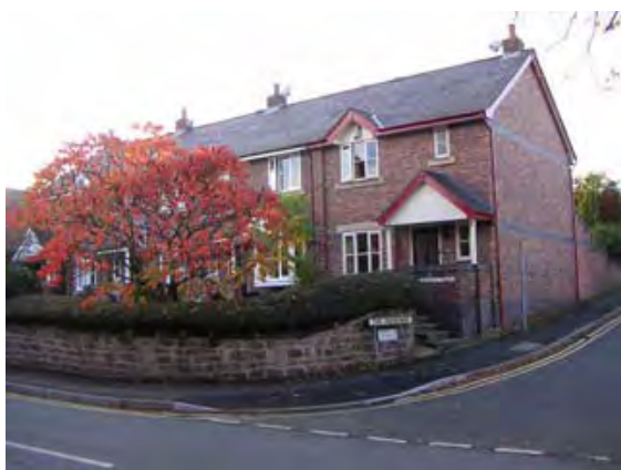
Cottages at entrance to The Ridgeway
