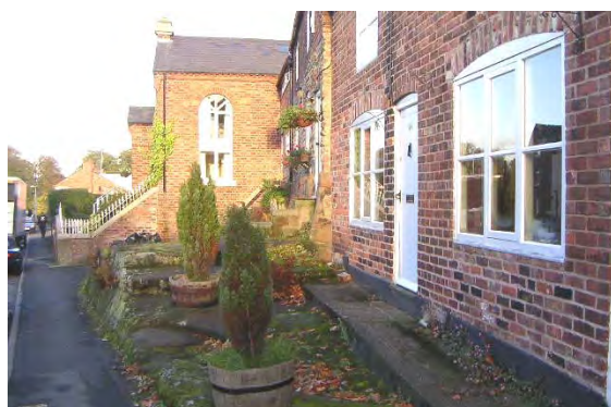
Cottages built on sandstone outcrop, Lower High Street
