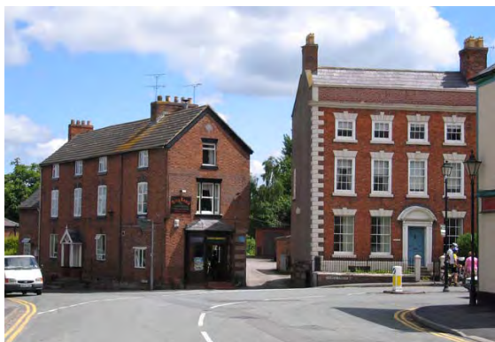
Three storey buildings in village centre [The Flaggs and King Louis Fish and Chip Shop]
