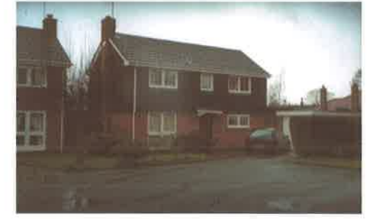
Similar house without extension
