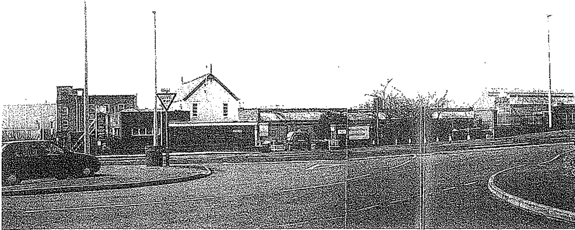
Photograph 1 Main Entrance from A56 Chester Road
